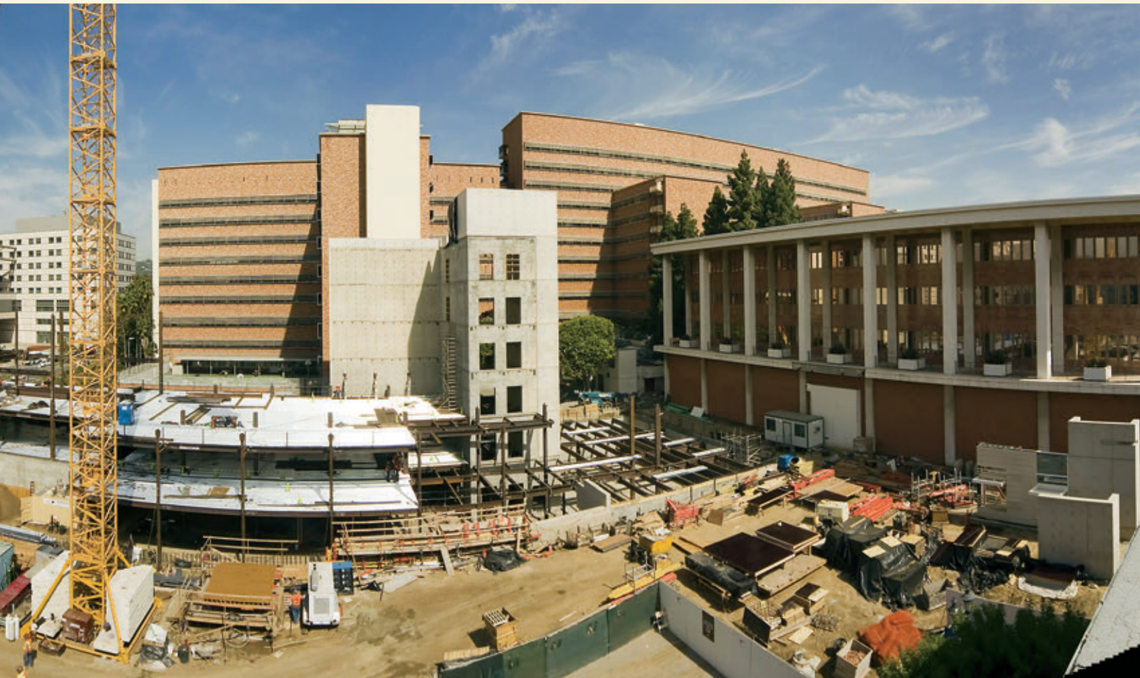
Wasserman Building construction site, October 14, 2011
