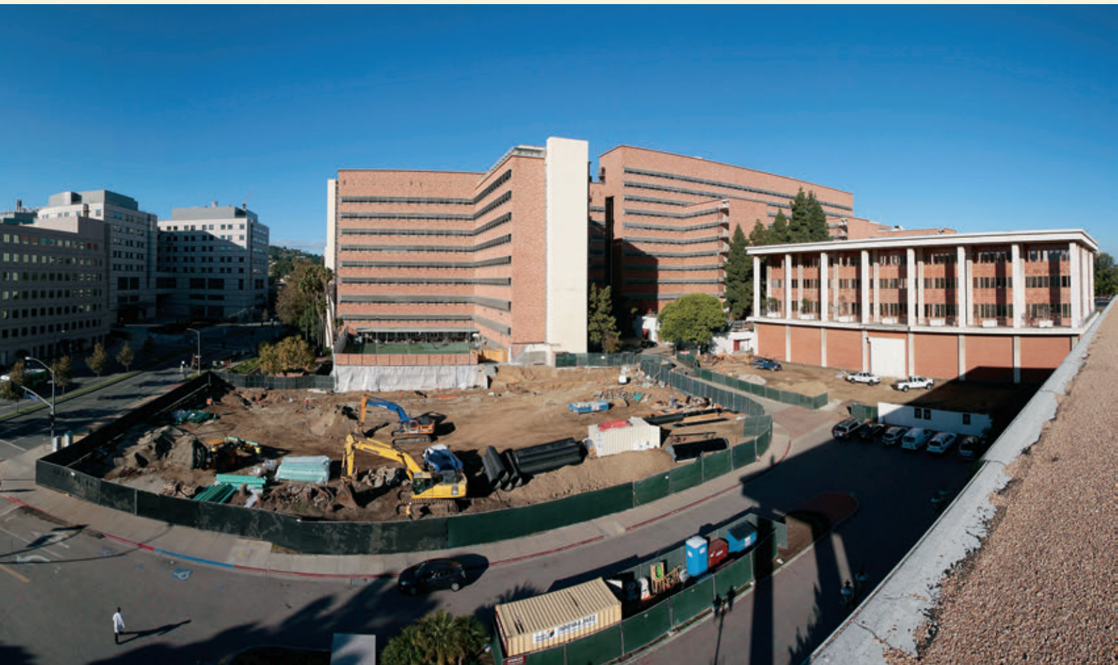
Wasserman Building construction site, November 22, 2010
