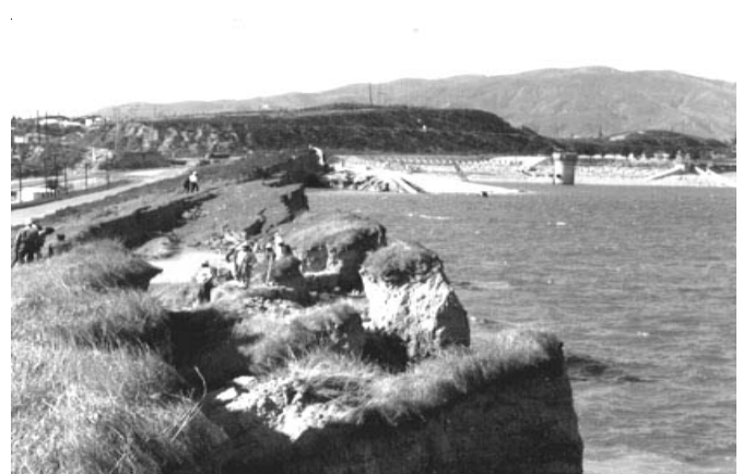
Figure 41 - Lower San Fernando Dam that was badly damaged by the 1971 San Fernando Earthquake.
