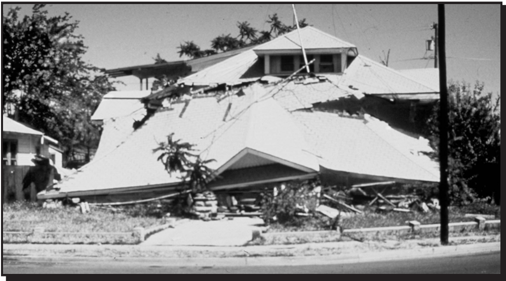
Additional damage from aftershocks
