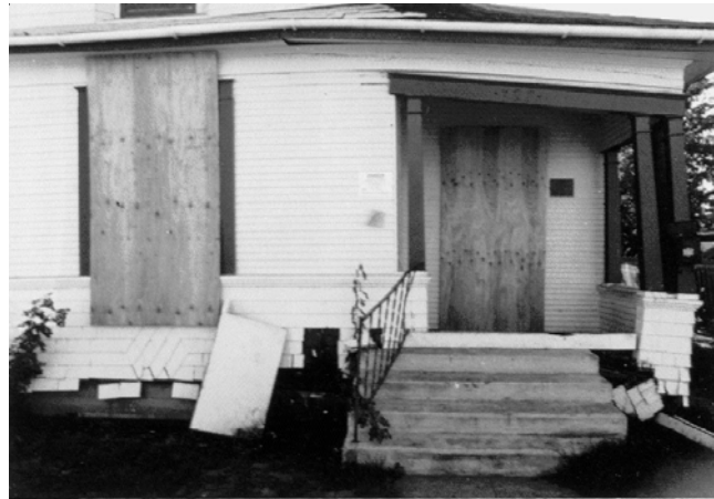
Office of Emergency Services
