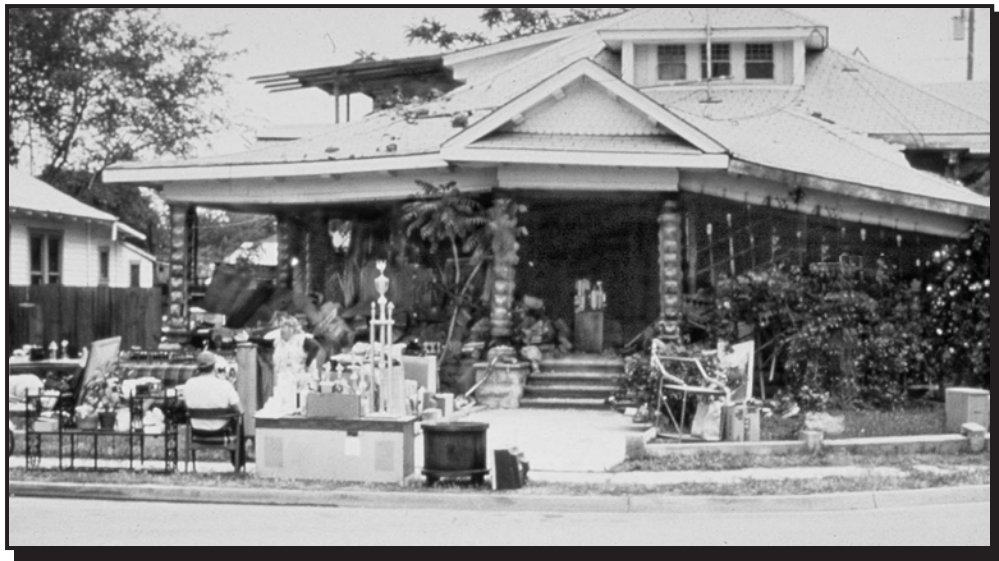
Damage from magnitude 6.7 earthquake
